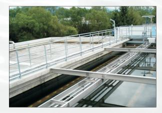
sedimentation tank from which separated activated sludge is routed to the regeneration tank. Excess activated sludge is removed with pumps to the sludge management
